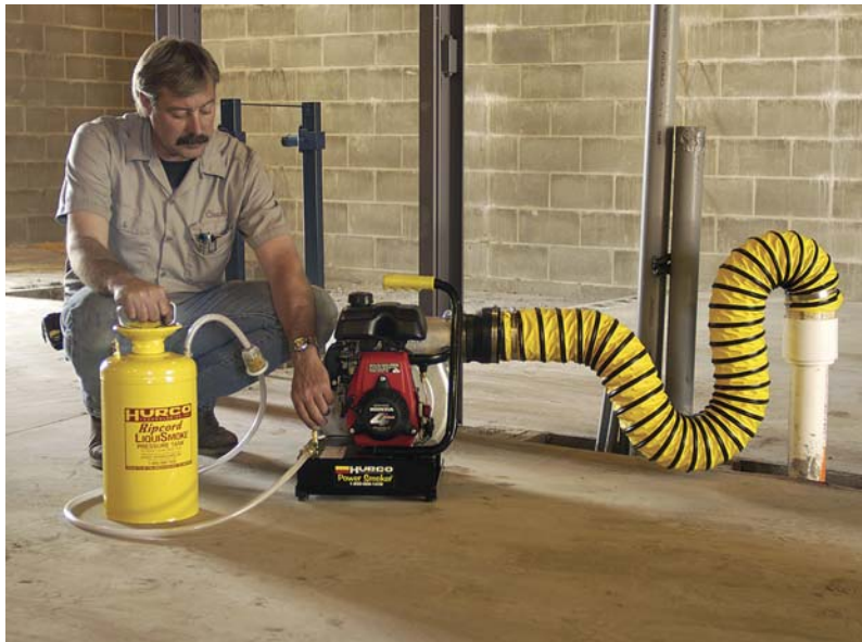
Typical set up for Smoke Testing
