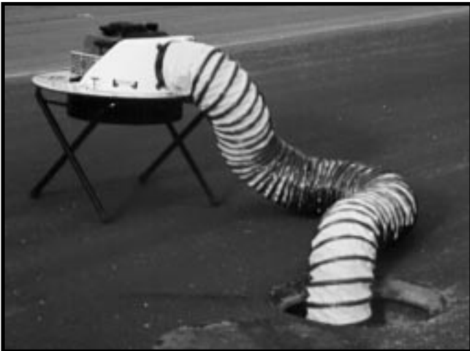
RIPCORDER assembled for blow-in ventilation
