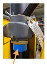
**Vacuum Relief Valve** – Located on Air Filter Tank.
