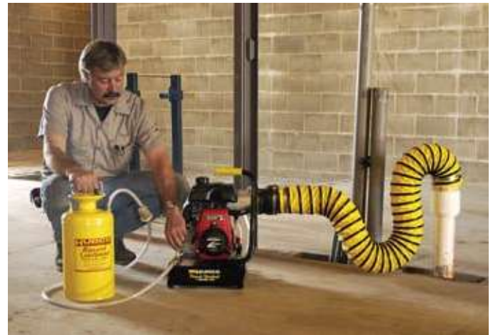
Typical set up for Smoke Testing
